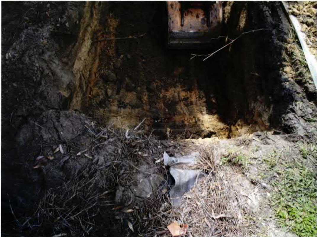
Picture 2: UST 1294Eagle removal in progress.
